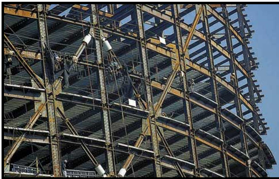
Figura 10. Torre Mayor – México
