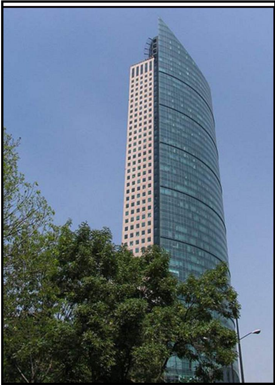
Figura 11. Torre Mayor – México
