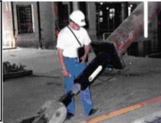
Figura 5 Dampers in chevron braces
