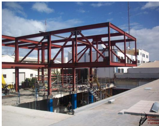
Figura N°92: Arriostre Diagonal
