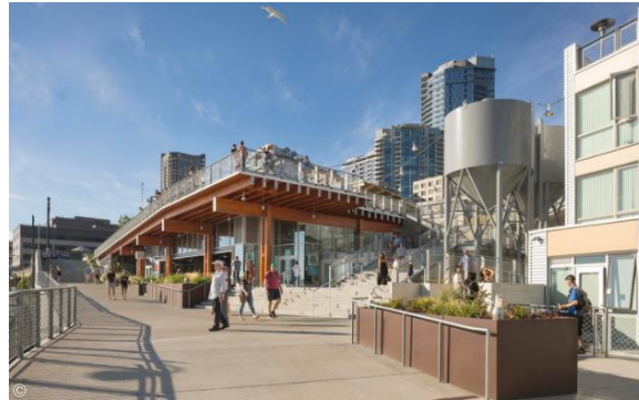
Figura 12: Fachada Pike Place Market Front
