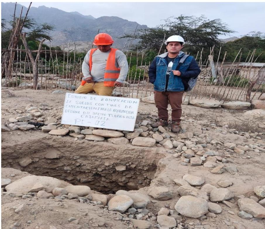
**Fotografía 04***Excavación de calicata C-03*
