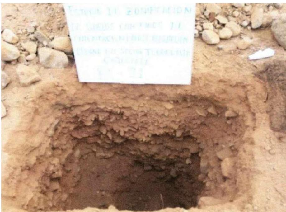
**Fotografía 03***Excavación de calicata C-02*
