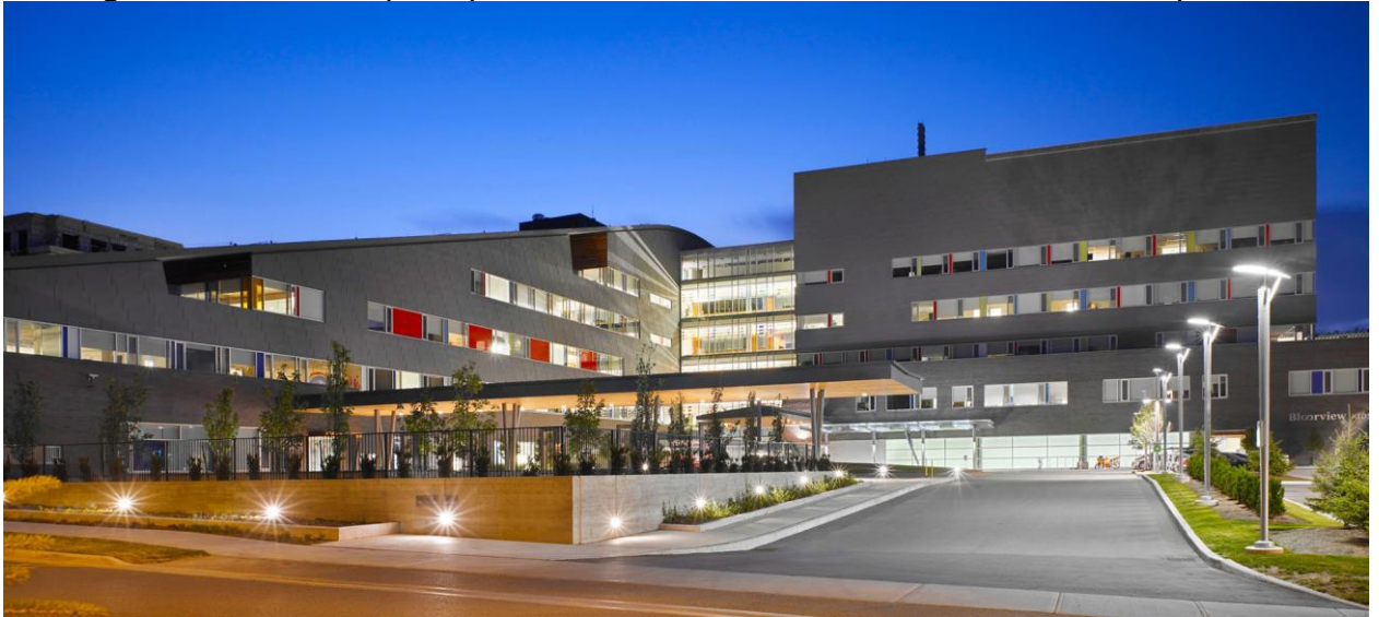
Figura 82: Fachada principal Holland Bloorview Kids Rehabilitation Hospital
