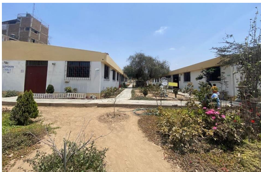
Figura N°17: “Instalaciones exteriores, C.S.M.C.”
