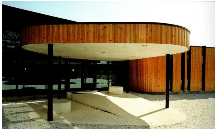
Figura 55. Ingreso al Oslo International School
